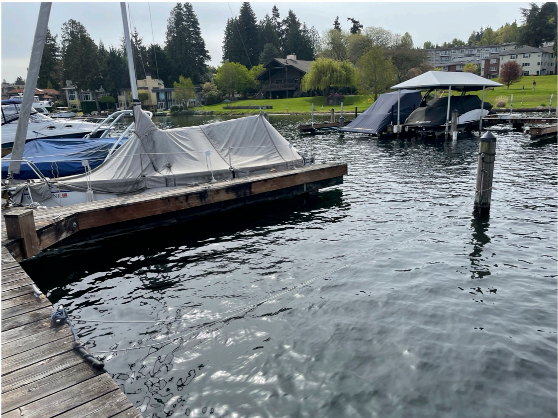
Photo 4 - Barneson slip existing conditions.
