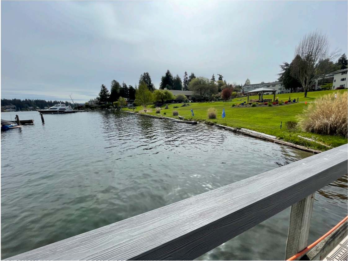
Photo 5 -Shoreline conditions east of marina.
